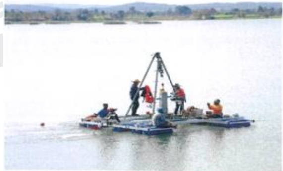
Fig 25 Installation of water level monitors in reservoirs
